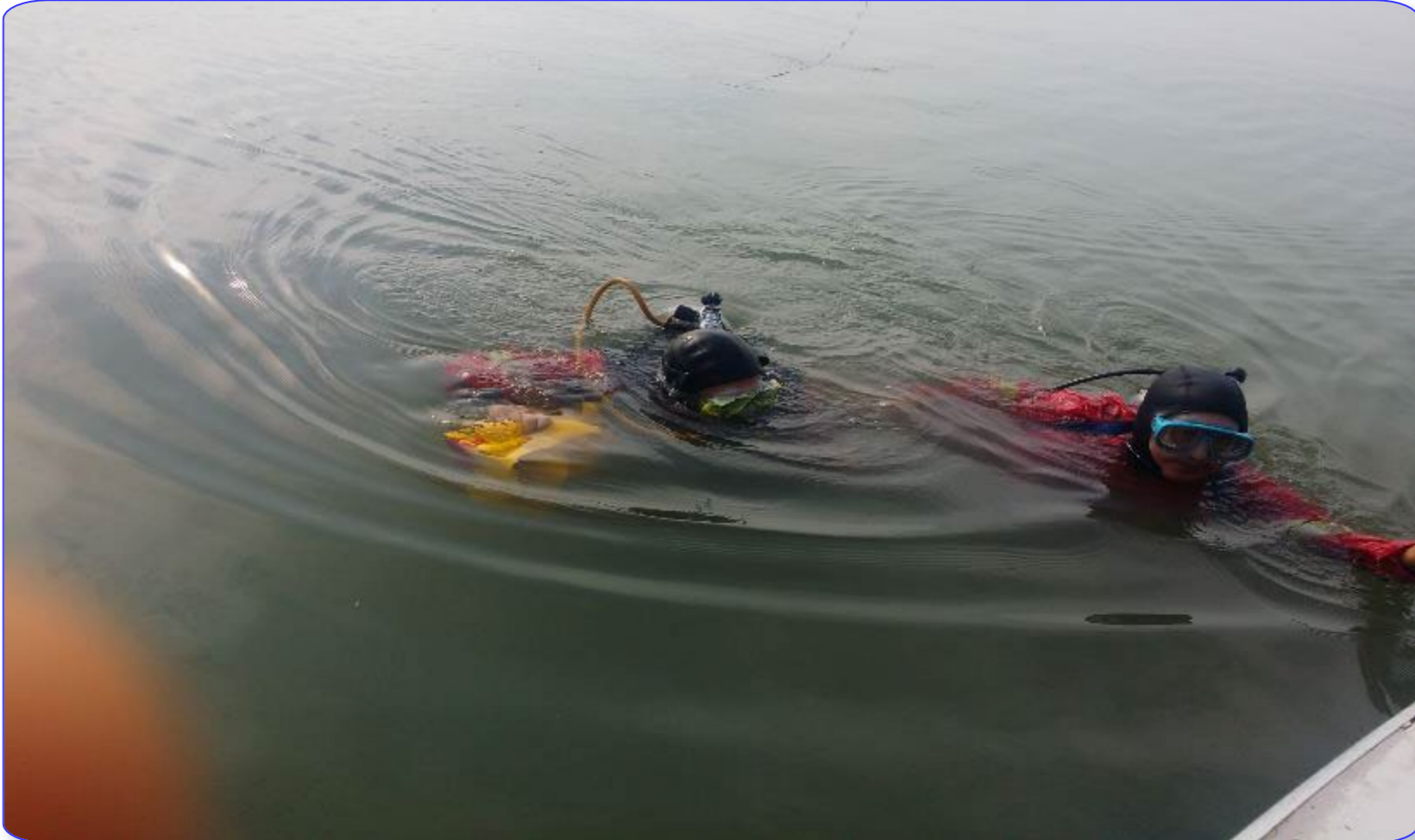
CURRENT MONITORING ADCP Installation
